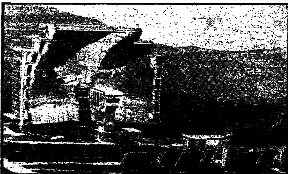
The solar furnace at Odelle in the French Pyrenees. The movable mirrors (foreground) reflect solar radiation on the giant parabolic mirror, which focuses the rays on the furnace located in the white tower
